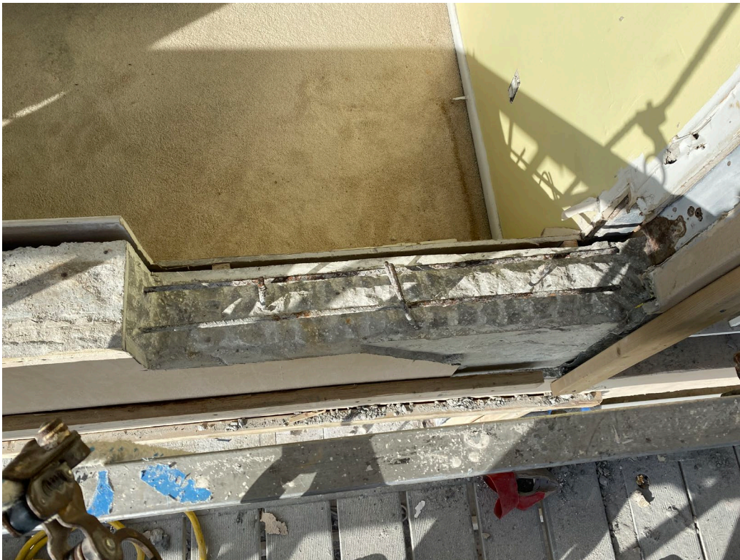
Picture 4: Unit 204 window sill repair
