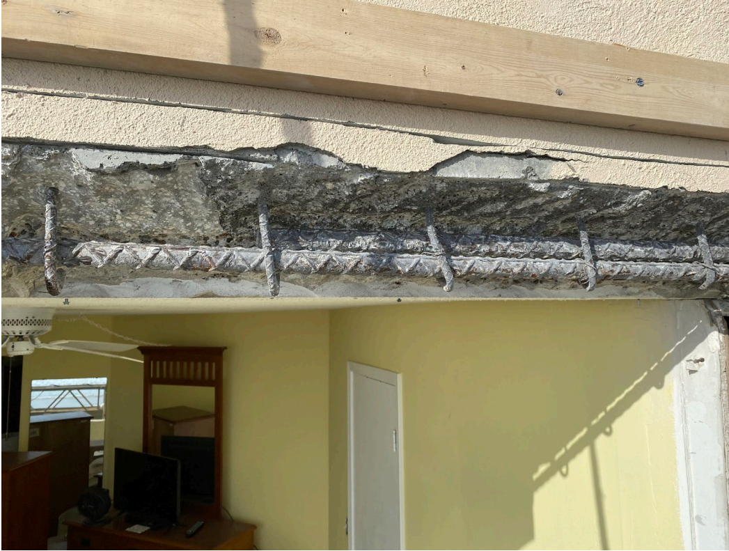
Picture 5: Unit 204 header repair
