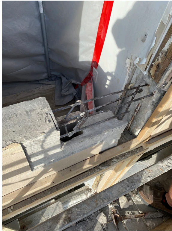
Picture 3: Unit 203 window sill repair
