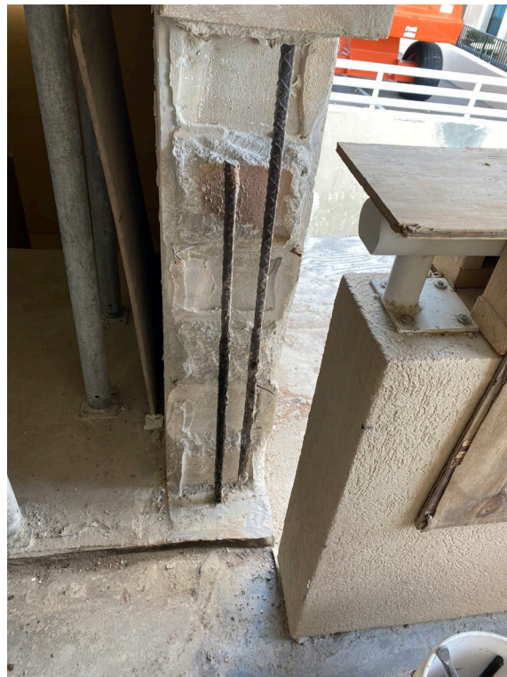
Picture 2: Typical jamb repair on North stairwell
