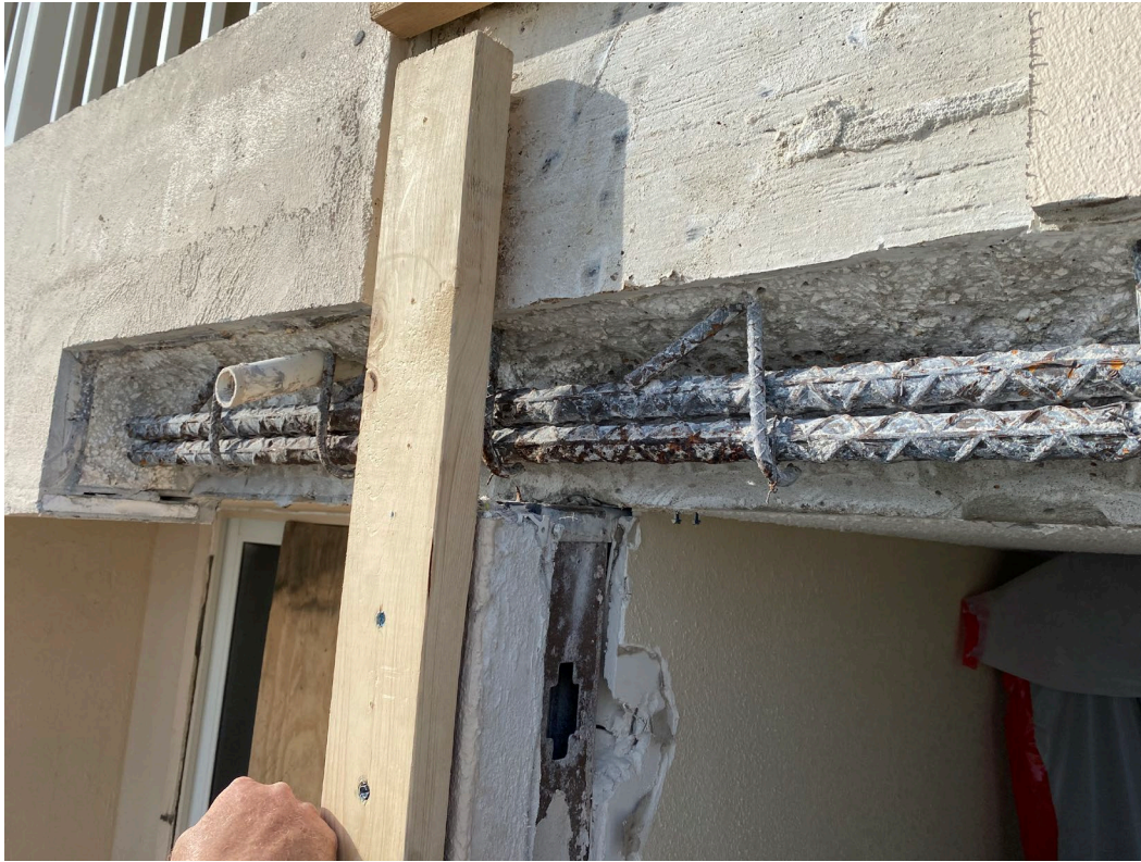
Picture 7: Unit 105 header repair
