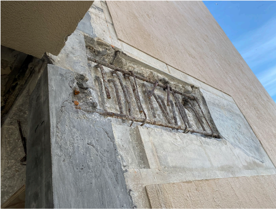
Picture 1: Wall repair on North stairwell
